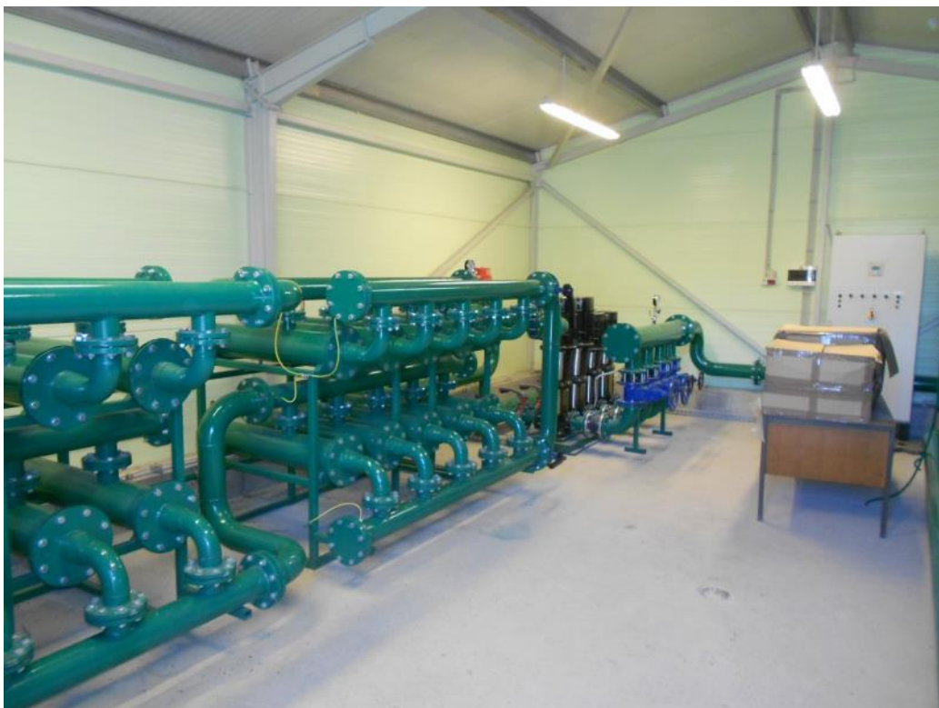
Figure 30: Fibre filters for waste thermal water before being reinjected into Le-3g well in Lendava geothermal district heating system, Slovenia
