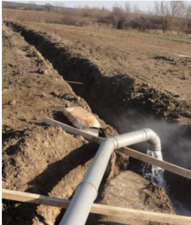
Figure 29: Discharge of cooled geothermal water (30 °C) into a melioration channel in Bošnjaci (Croatia) where the thermal water is used for heating of greenhouses
