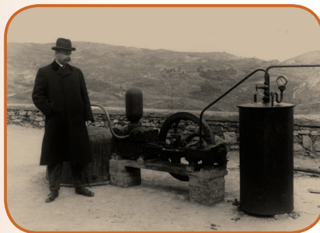
Figure 2: The world's first geothermal power station with a 10kW generator in Larderello dry steam field, Tuscany, Italy (Source: IGA)
