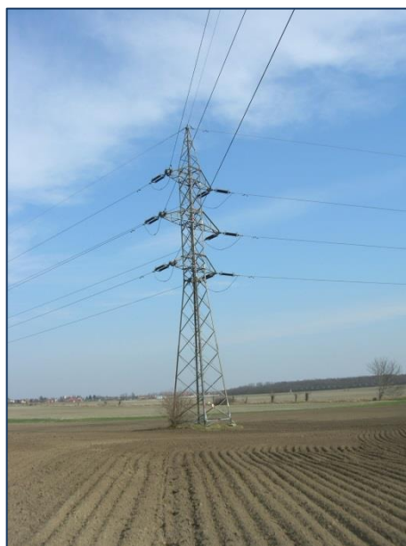
Pylons of 2x110 kV lines in Slovakia
