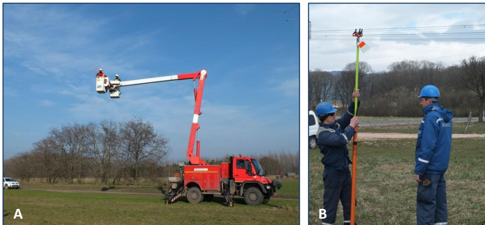
Fig. 25 The most used installation techniques of line marking: (A) bucket truck and (B) hot-stick
