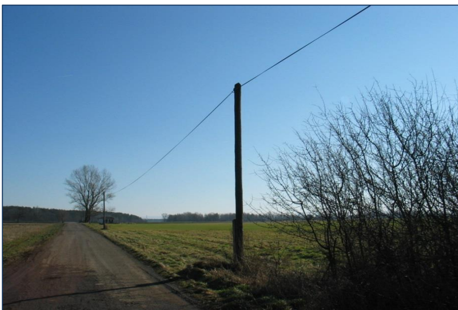
Fig. 4 Low voltage power line in one black cable design
