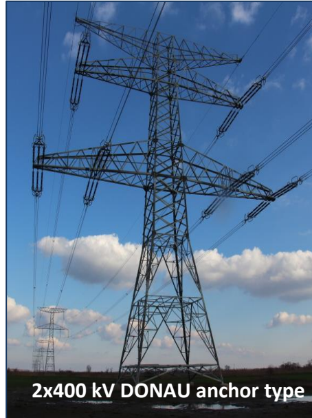
Pylons of 400 kV power lines in Slovakia
