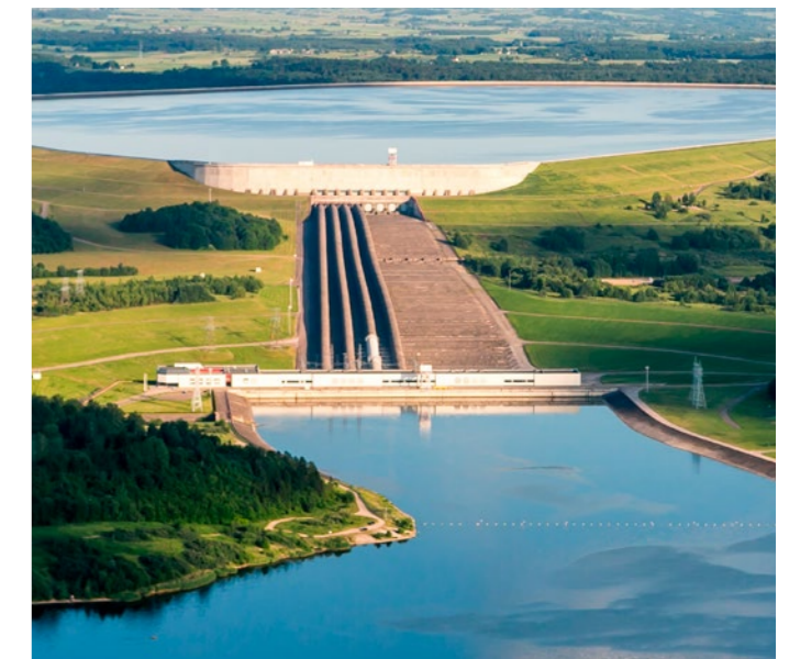
Fig. 5: Pumped hydro station
